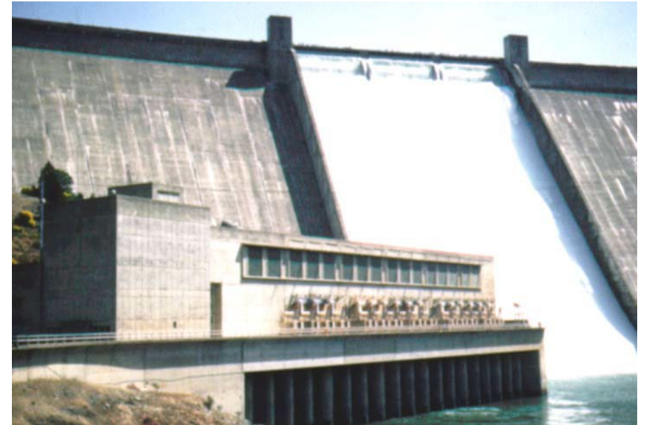
Powerplant at Shasta Dam
