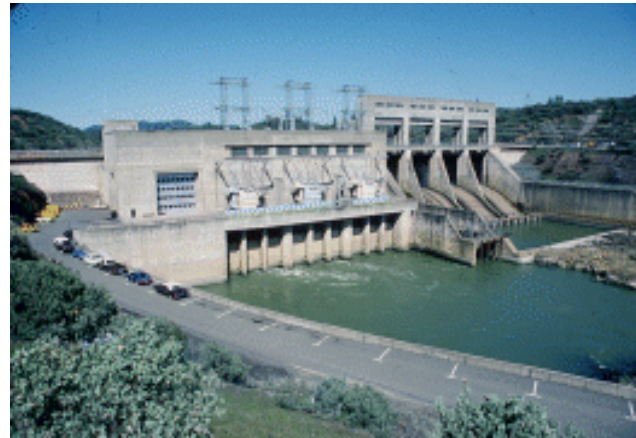
Keswick Dam and Power Plant
